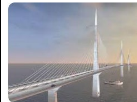
Qatar bridge links in with our Design Technology part of the topic, where we will be making our own bridges.
